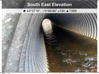
7' diameter corrugated metal pipe culvert. Note: bottom/invert of the pipe is in very poor condition.
